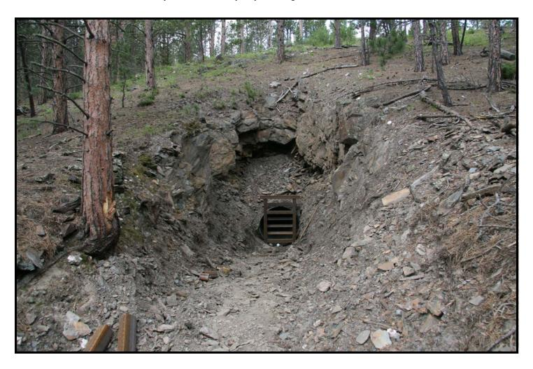
The Papcke's mine after the installation of the culvert and bat gate....
