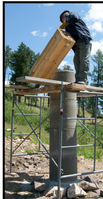
Interior: a modified stacking rocket box design was constructed from rough-sawn pine on a cedar base
