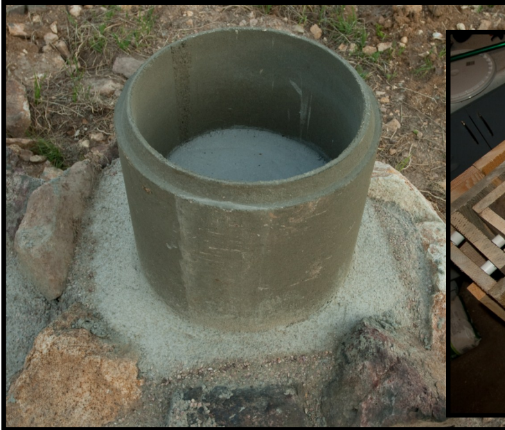
44 - 60lb. bags of concrete were used to build the foundation
