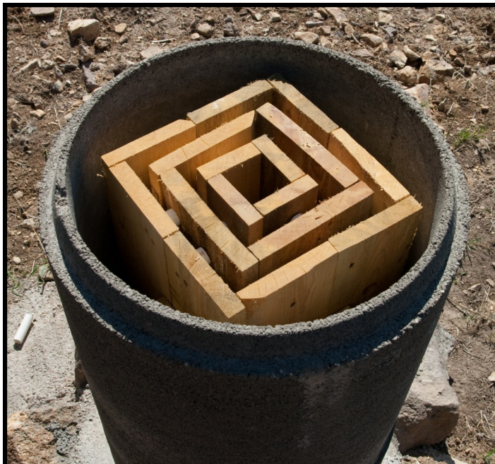
The first section is put into place...
